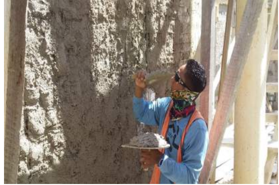
Plastering F5, B5
