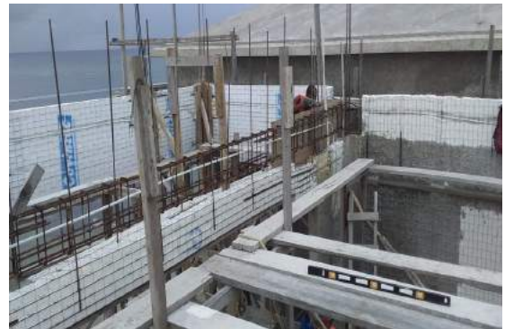
Installation of Coventec Wall Panels, Beam Rebar, Beam & Column
