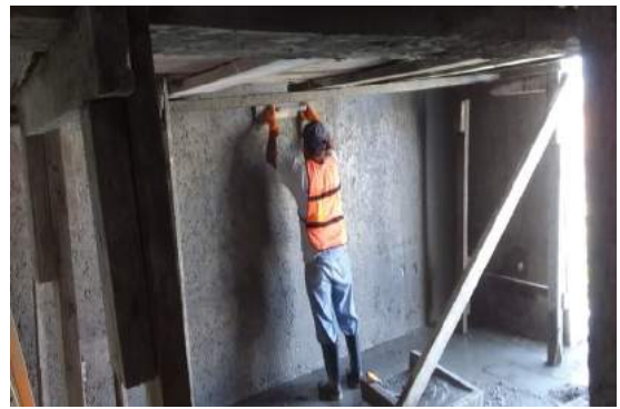
Plastering A, B, C Level 4
