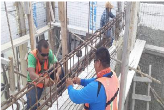
Installation of Coventec Wall Panels, Beam Rebar, Beam & Column
