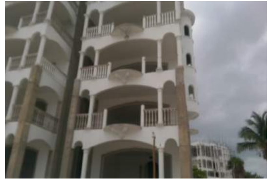
Installation of Handrails
