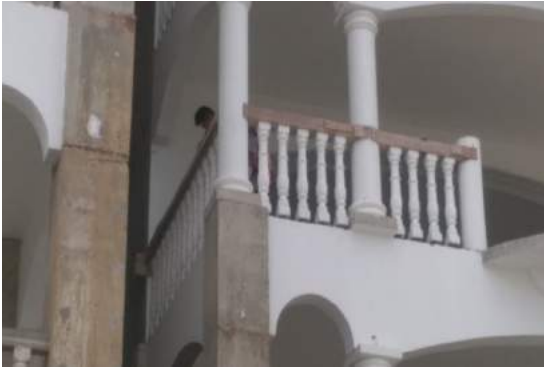
Installation of Handrails
