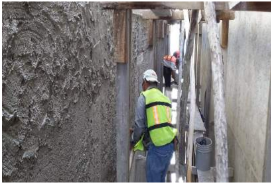
Plastering F5, B5
